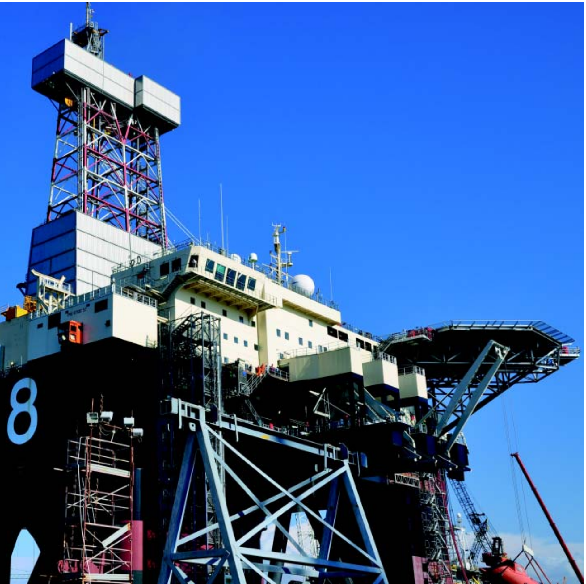
Cabins Module created by Navalimpianti for Scarabeo 8
