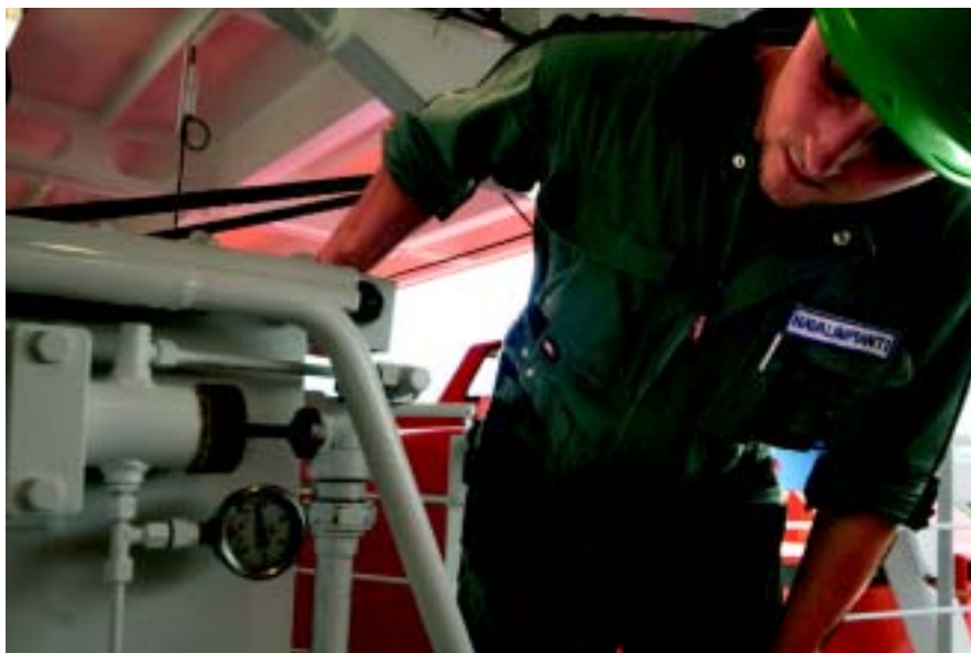
Navalimpianti Tecnimpianti service technicians checking operations
