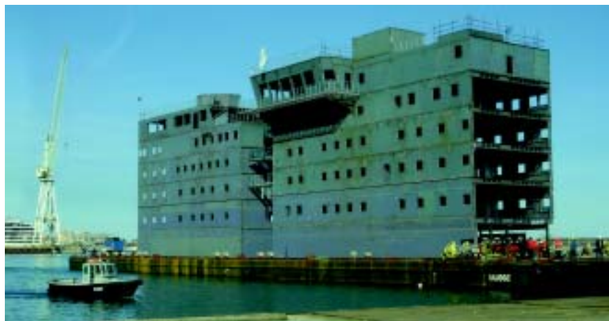
Cabins Module for Scarabeo 8 under construction
